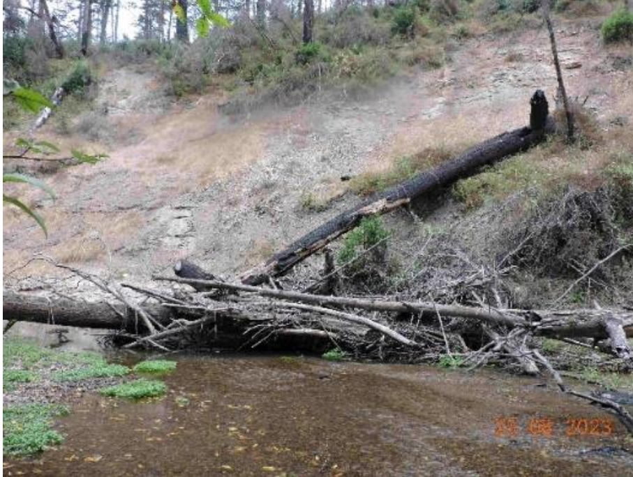
Photo 23. Mile 1.8, looking downstream. 2022 slope failure scarp and channel wood at the bend shown in photo 22.
