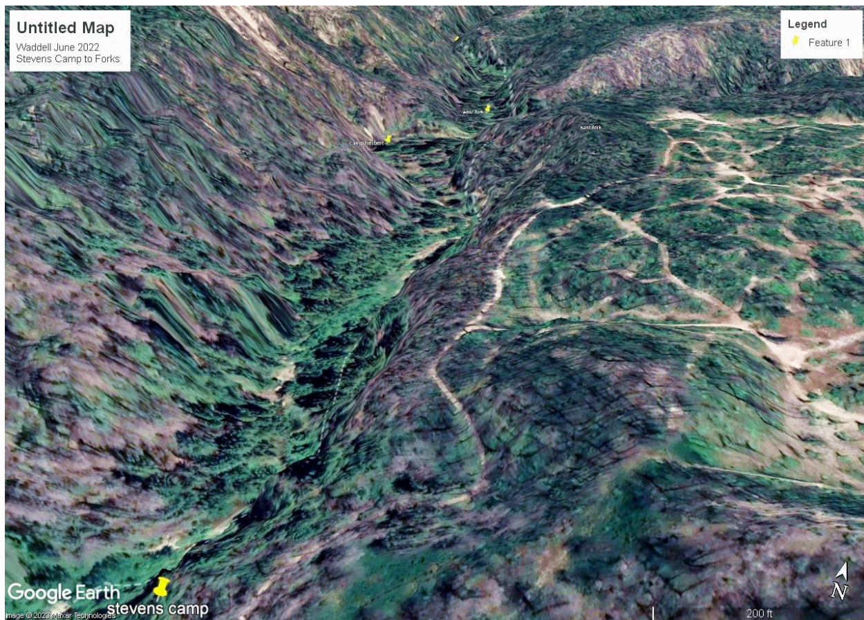
Figure 10. Google Earth aerial photo from 10 June 2022 between Stevens Camp (mile 2.55) and the East and West forks of Waddell Creek. In 2021 streambed sedimentation and pool filling extended from the forks downstream half way to Stevens Camp. In 2022, erosion from the west slopes of Waddell and West Waddell creeks extended streambed sedimentation downstream to at least mile 1.75 (Twin Redwoods Camp). The upper east slopes and hilltops between Stevens Camp and the East Fork (right in the photo) are private property that was salvage logged for redwood in 2021; the green is primarily blue blossom Ceanothus .
