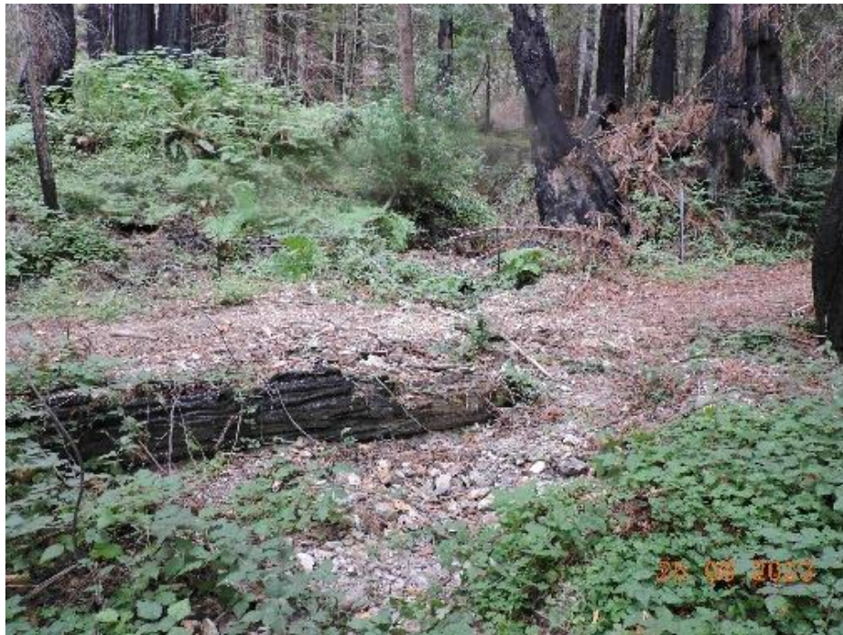
Photo 30. Mile 2.15, looking upslope across road. Seasonal drainage carried sediment and angular mudstone gravels across road and down to Waddell Creek in 2023.
