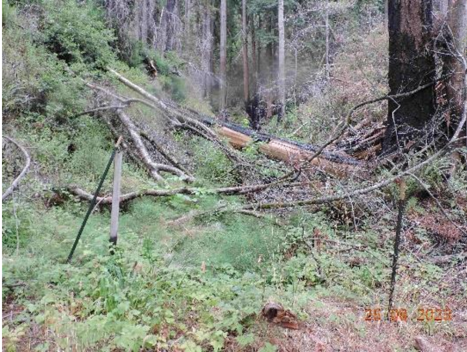
Photo 27. Mile 2.05. "Tramway Springs," a wet year perennial drainage upslope of the road.
