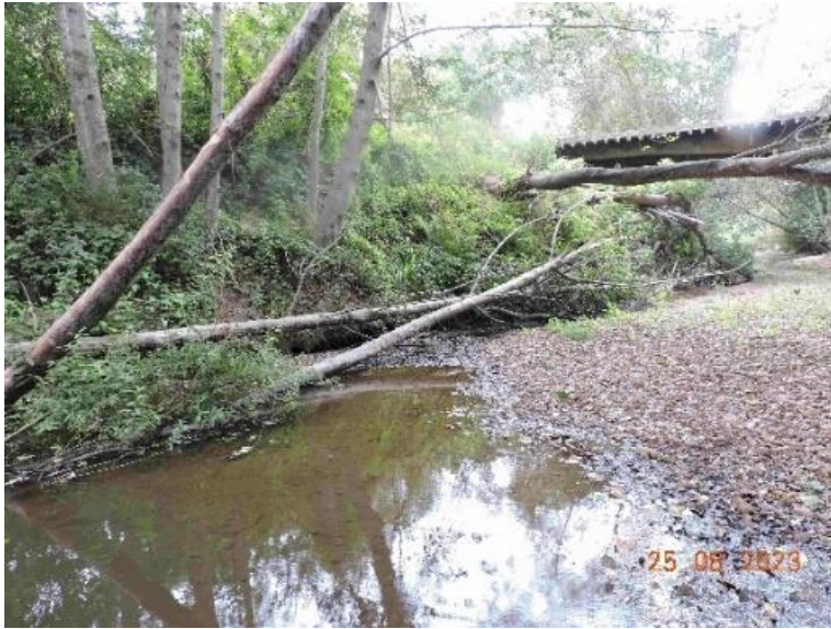
Photo 1. Mile 0.65 (from Highway 1). Looking downstream to the bridge above the lagoon. Winter 2023 flows reached to the bottom of bridge several times and flowed through the flood plain with wood to agricultural fields on the left bank. Streamside alders were toppled and the channel widened and flattened.
